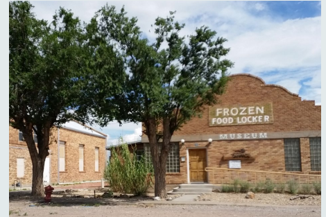
Siberian elms in front of the former Carrizozo Ice Plant. Photo Credit: Jennifer Dann, NMSF
