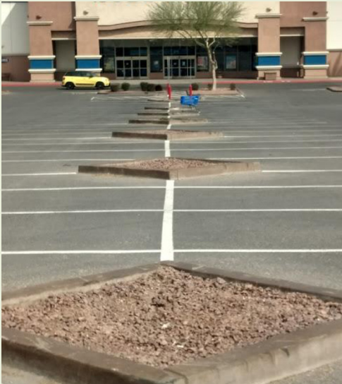
Parking lot in Las Vegas demonstrates the lack of trees and shows that there is work to be done. Photo Credit: Lisa Ortega.
