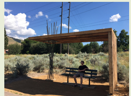
Shade shelter utilizes reclaimed wood and locally-sourced materials. Photo Credit: Climate Smart Missoula.
