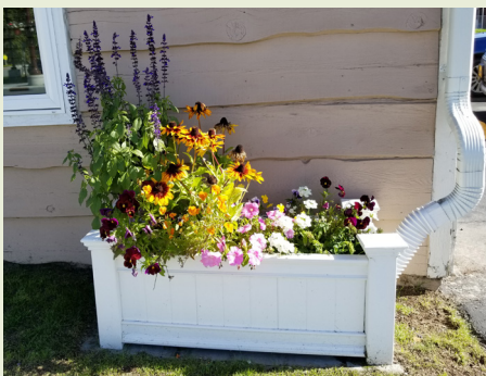
S Salon is using green infrastructure such as flow-through planters to help retain rainwater and soak it into the ground on their property. Photo Credit: Alaska DOF.
